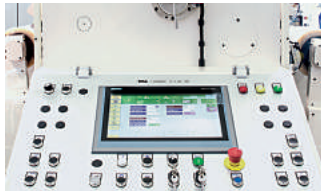
Main operating panel.
